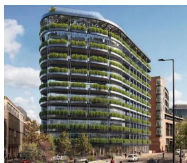
40 Highborn Viaduct - before & after
